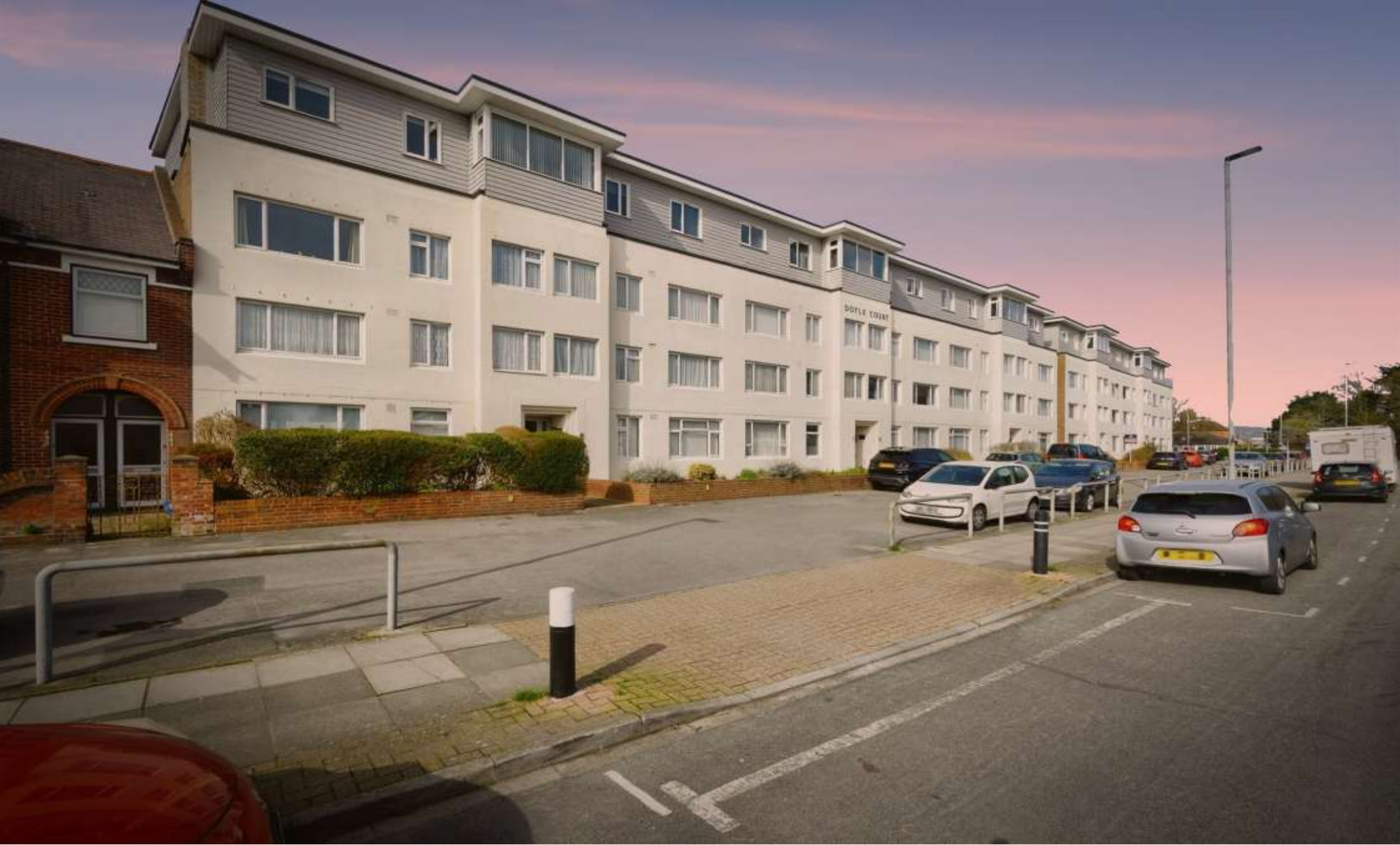
Doyle Court London Road, PORTSMOUTH PO2 9HP
