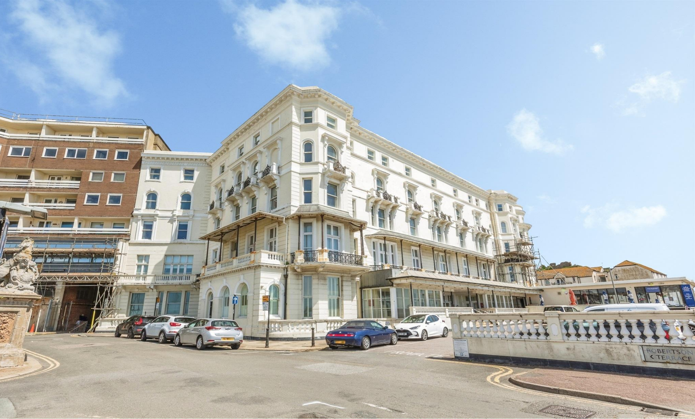
The Queens Apartments - Robertson Terrace, Hastings TN34 1JN
