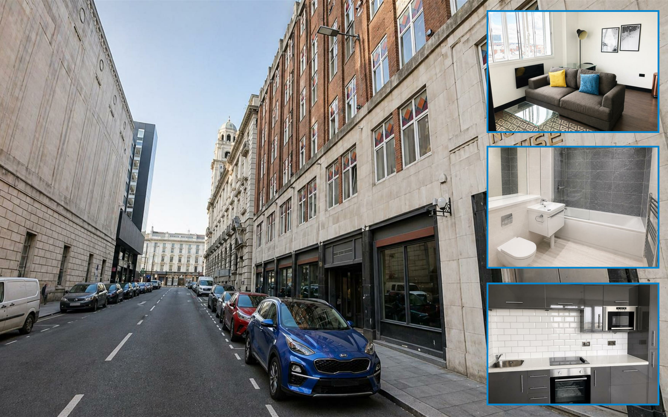
North House 17 North John Street, Liverpool , Merseyside L2 5AA Auction Guide £70,000
