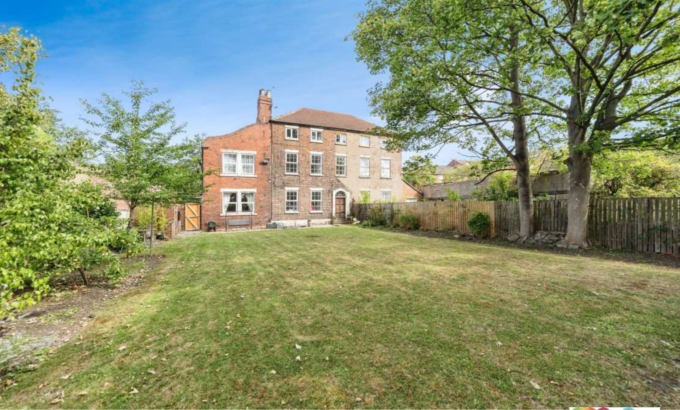
Wentcliffe House, Station Road, Ferrybridge Knottingley WF11 8NJ
