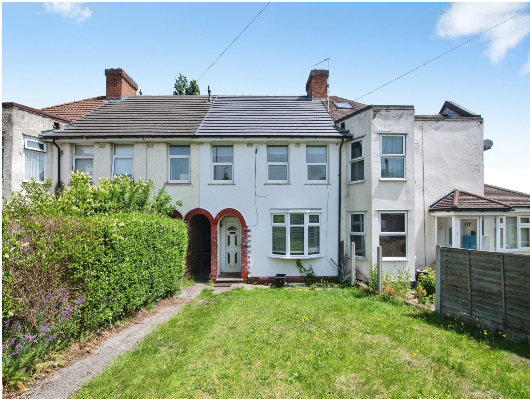
Cranbourne Road, Birmingham B44 0DE
