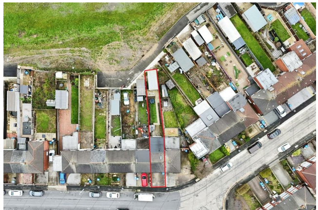
Aerial view of the property
