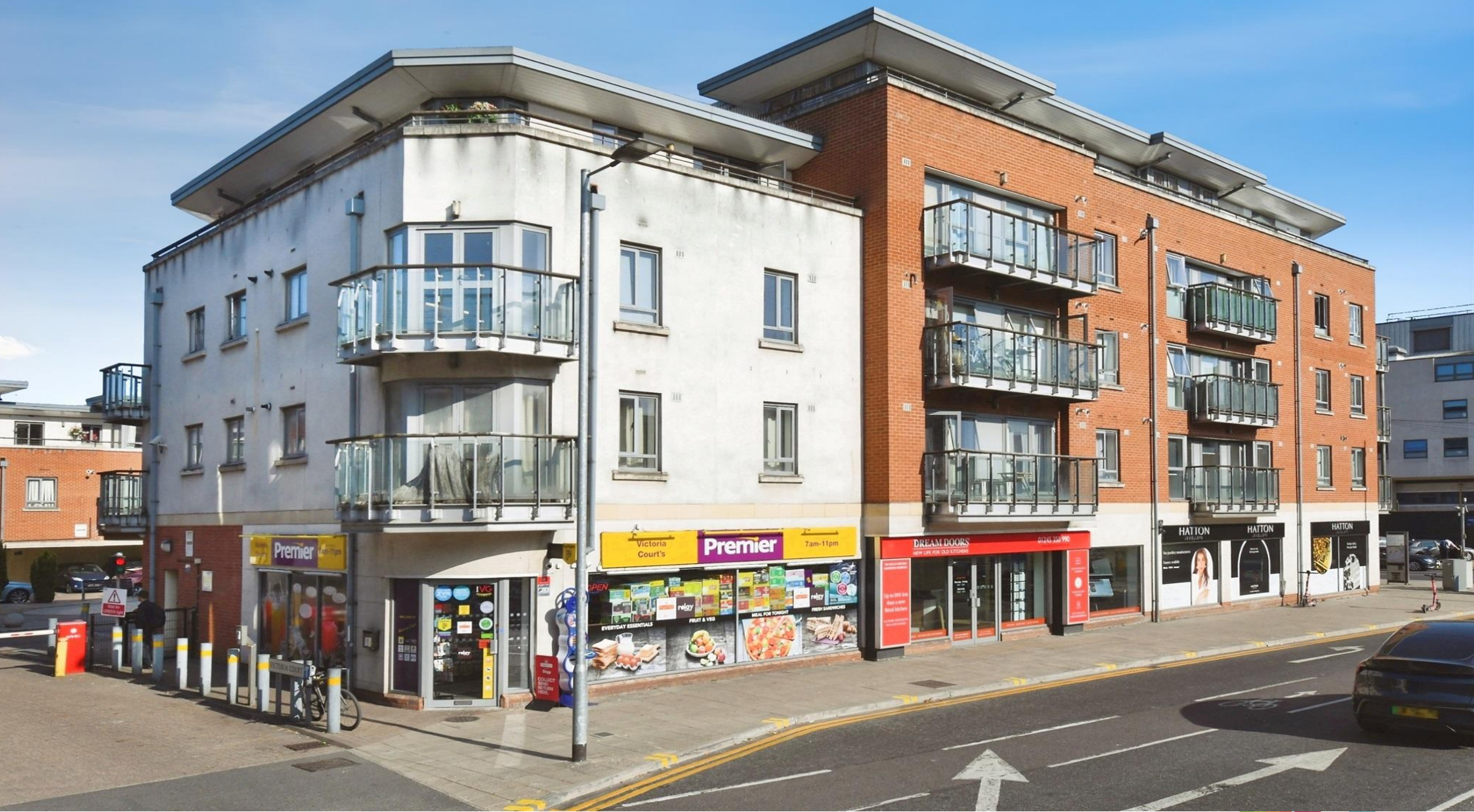
Victoria Court, New Street, CHELMSFORD CM1 1GP
