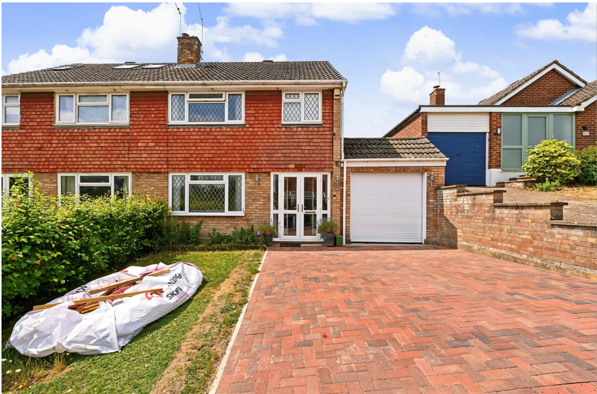
Abstacle Hill, Tring HP23 4DA
