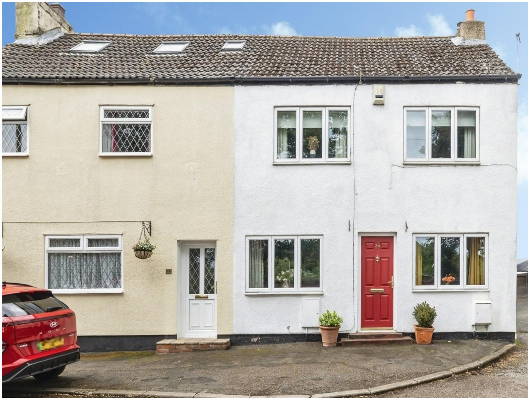
Riverside, Rawcliffe GOOLEDN14 8RN
