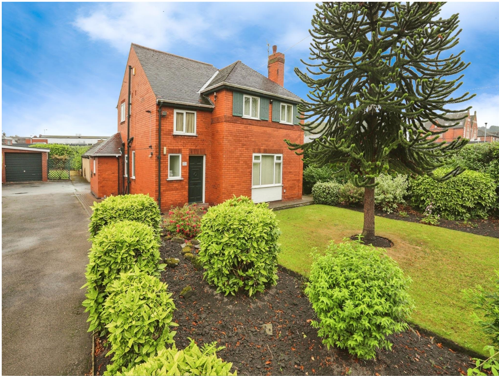
Ferrybridge Road, Castleford WF10 4JL
