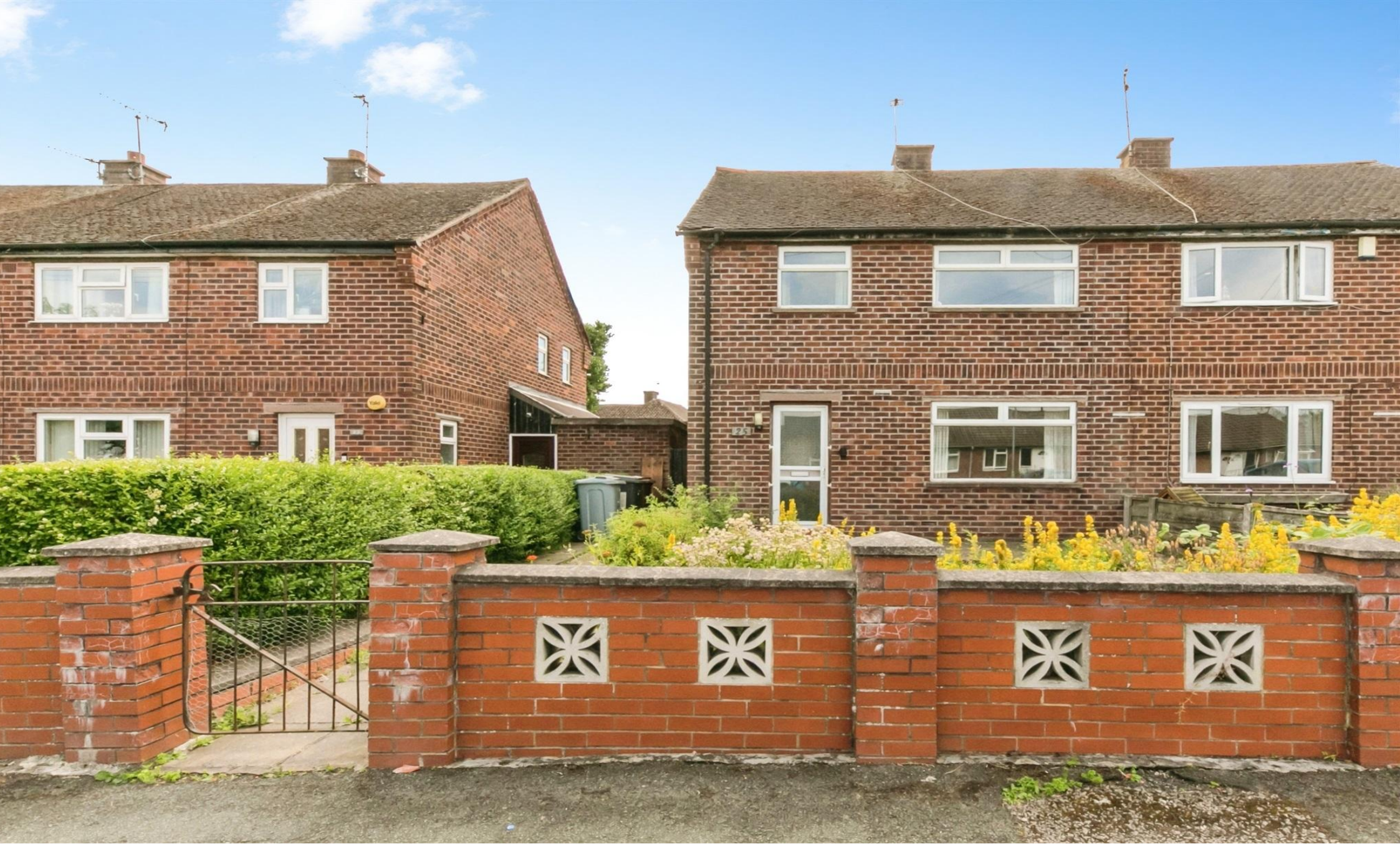
Queens Drive, Middlewich CW10 0DG
