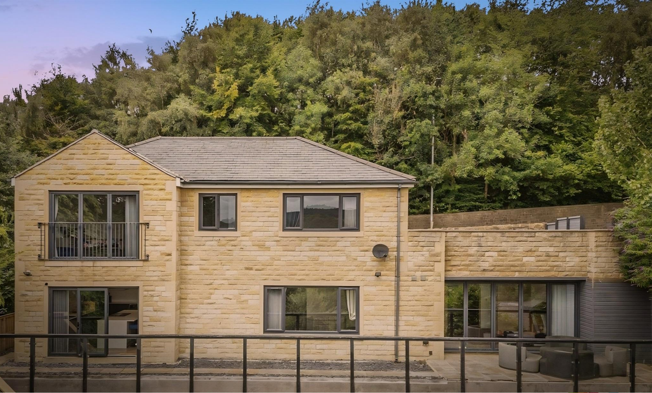
Valley House The Meadows, Sowerby Bridge HX6 2UN
