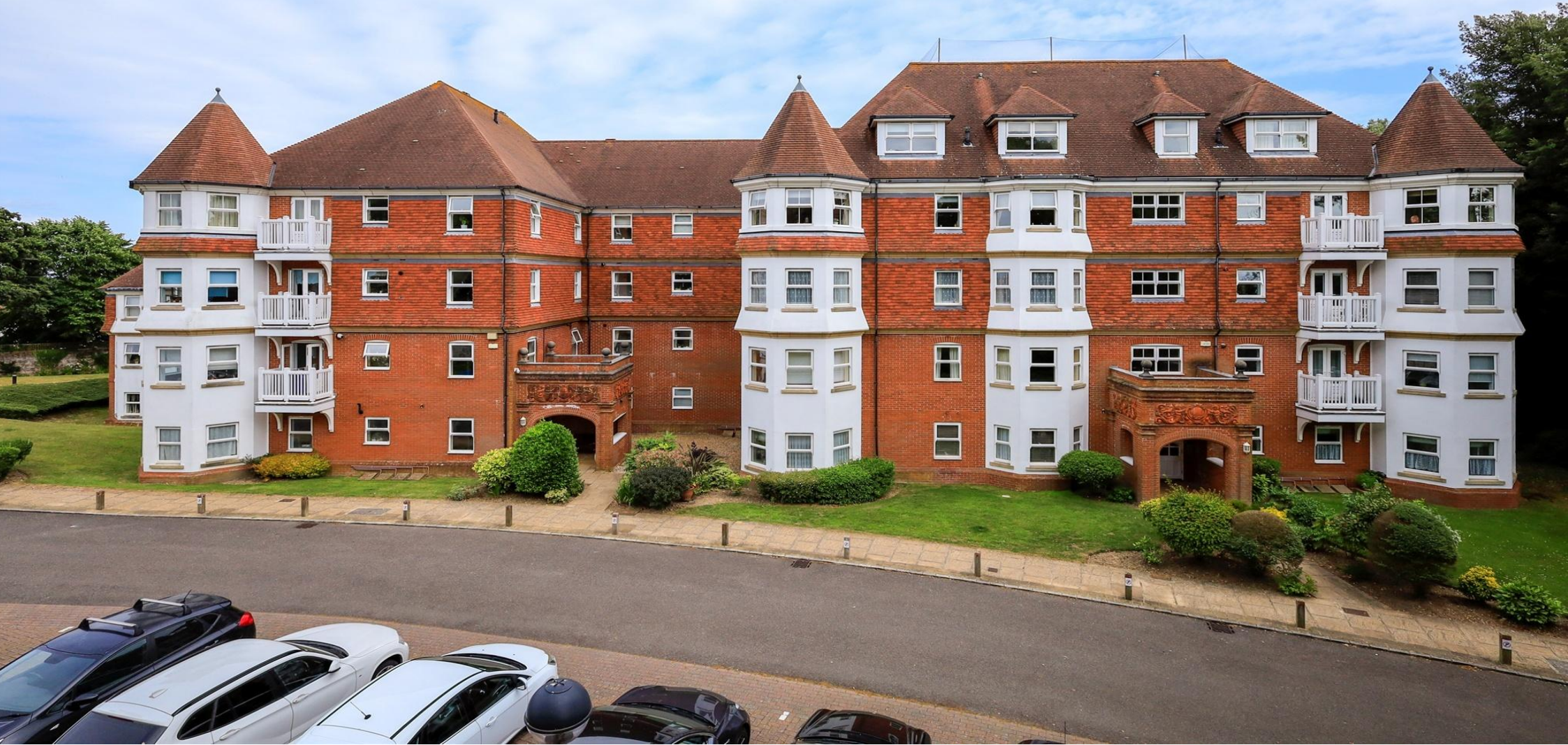
Eversley Court St. Annes Road, Eastbourne BN21 2BS
