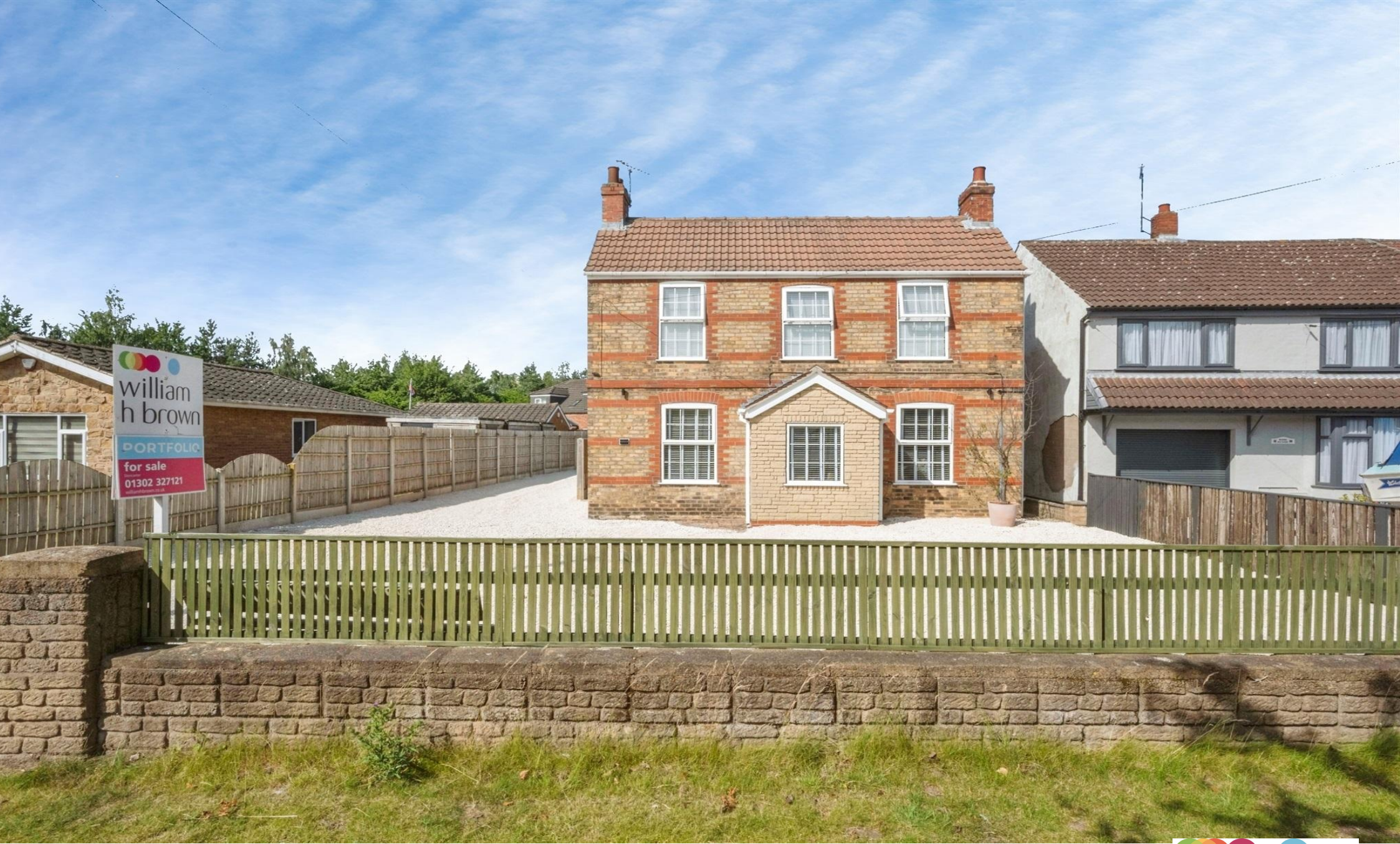
Gate House Lane, Auckley Doncaster
