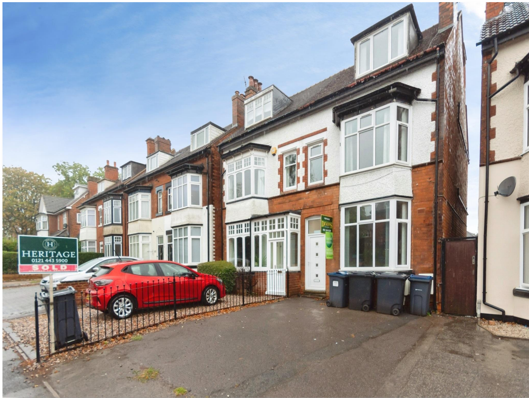
Alcester Road South, Birmingham B14 6DE
