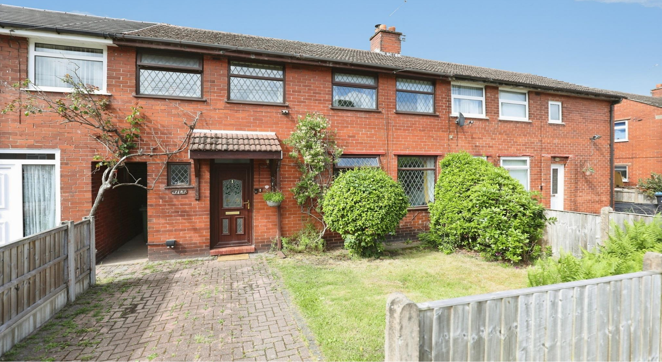
Farm Road, Weaverham Northwich CW8 3PG
