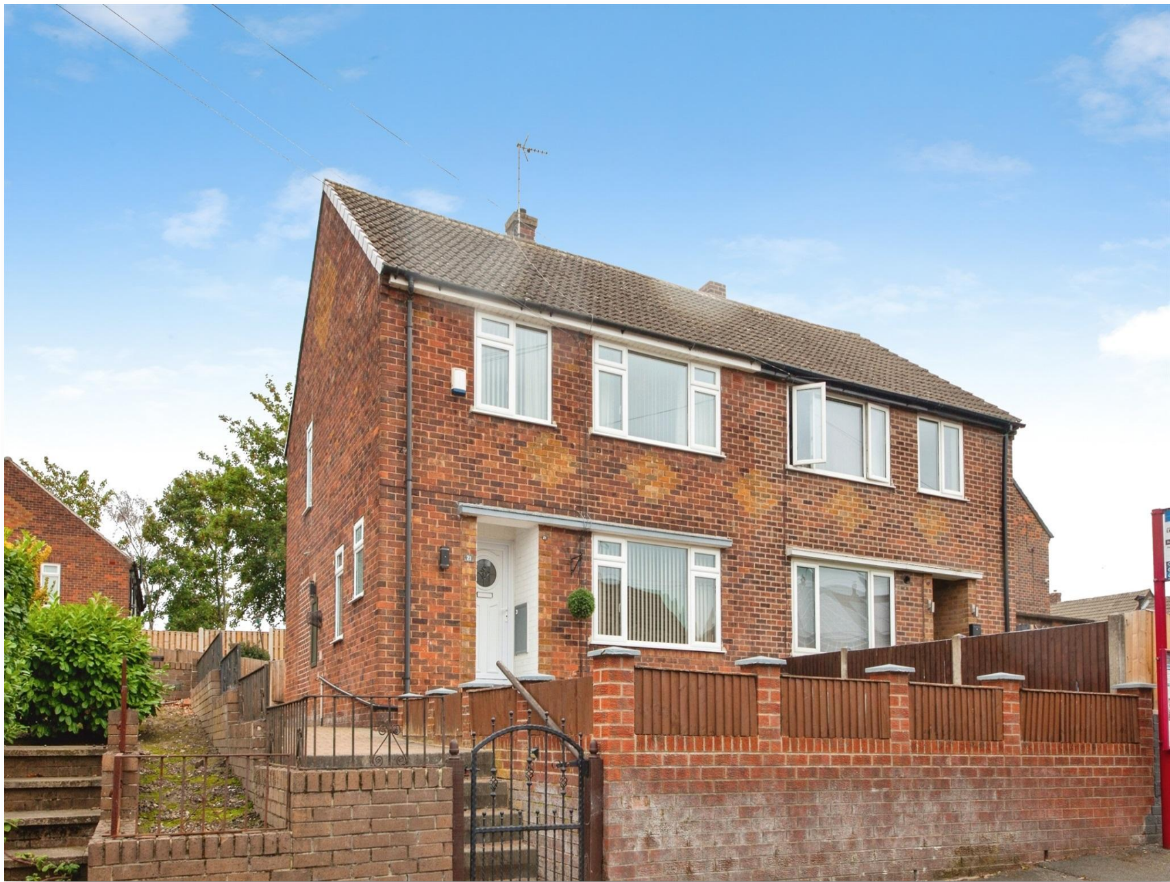
Ashfield Road, Hemsworth Pontefract WF9 4RN
