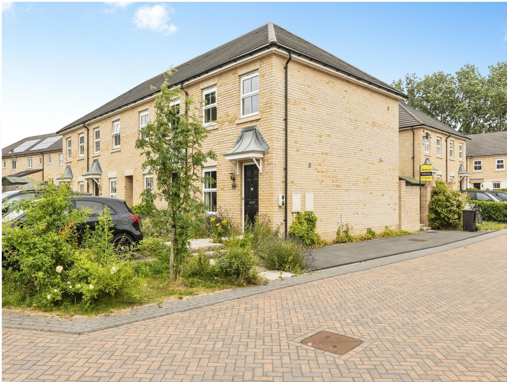
Castle Hill Close, Garforth Leeds LS25 2QE
