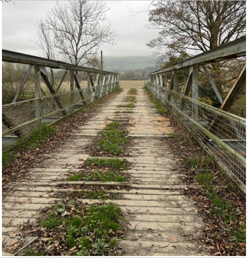
Bridge that runs over the river severn.
